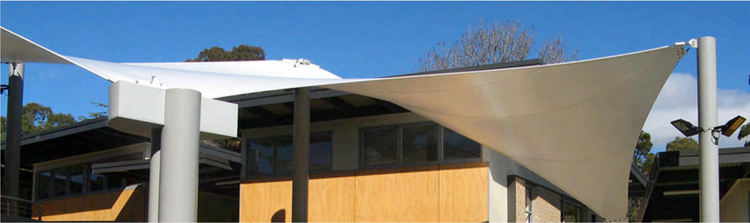
Tension shade membrane over Student Courtyard
